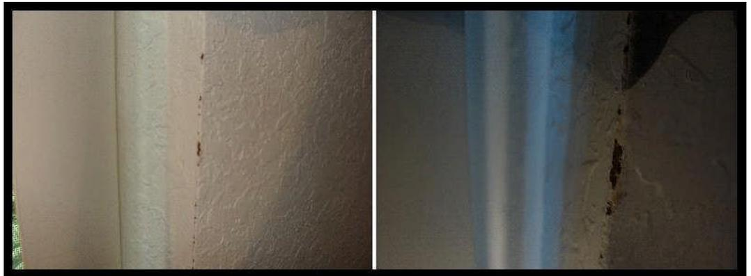
The left photo is of rusty corner molding under paint, the rust is expanding and bursting through the walls paint.
