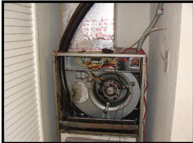
The photo is of the interior of the AC unit. Note black corrosion on the refrigerant lines on the left.
