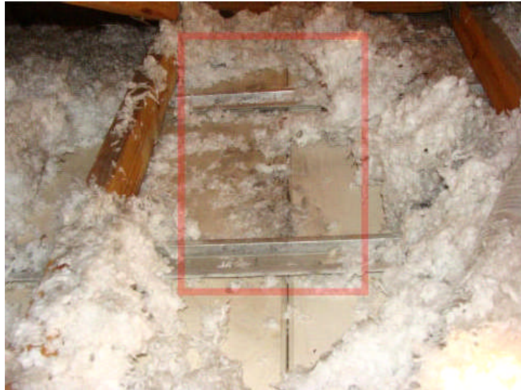
The above is a photo of mold under insulation in the attic above the stained closet.
