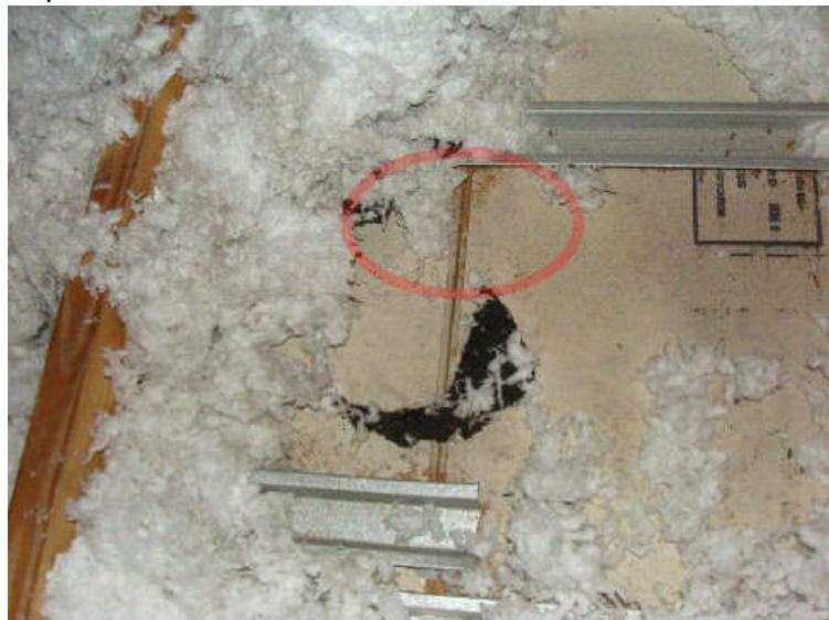
The above is a photo of mold under insulation in the attic above the stained closet.
