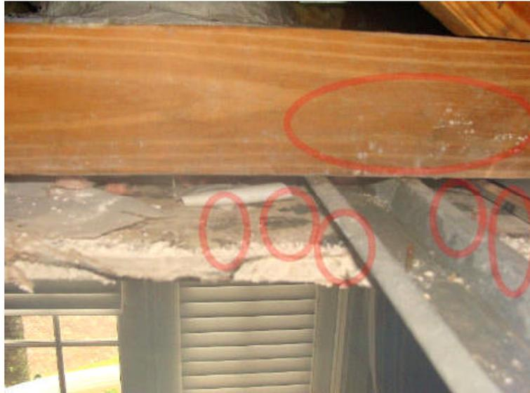
Note mold on the floor of the attic as observed from inside this ceiling hole.
