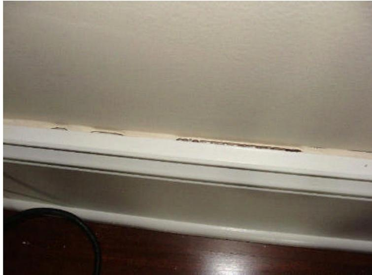
The above is a photo of the baseboard separating from the bottom of the wall in the first photo above. This is evidence of moisture in this wall.
