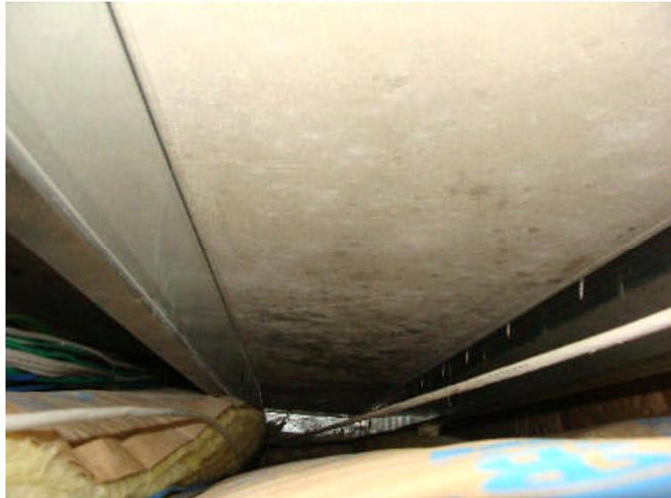
The above is a photo of mold inside the wall as viewed from inside the attic by looking into the hollow openings at the top of the wall.
