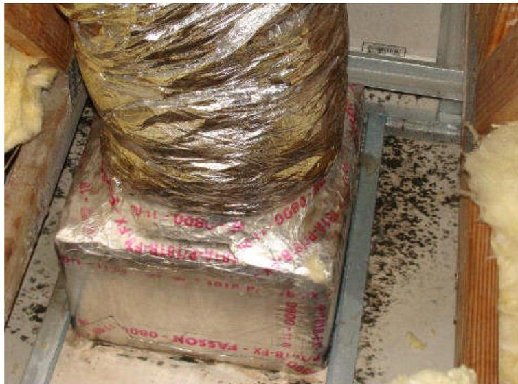
In several areas mold was around leaky ducts in the attic. Leaky ducts caused negative pressure in the home that pulled humid attic air into the cold walls below. The mold around many ducts is all the proof needed to prove beyond a reasonable doubt that the ducts were leaking cold air.
