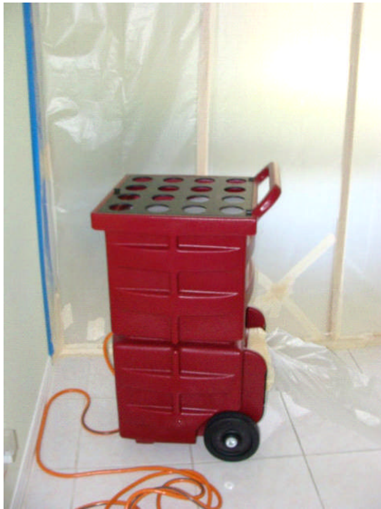
The above is a photo of containment and an air scrubber.
